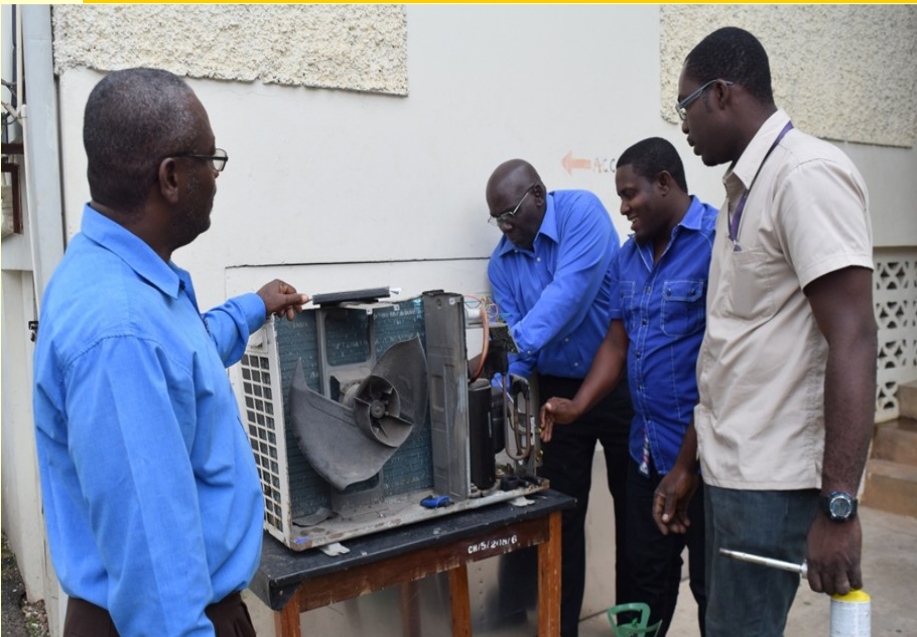
Heart Trust/NTA Lecturer, Mr. Roger Gordon (left) supervises the process of removing a defective compressor from an air conditioning unit by trainees, (l-r) SRHA Maintenance Manager, Mr. Richard Copeland, AC Technician from the May Pen Hospital, Mr. Dwight McLeod and AC Technician, Mr. Gary Smith from the Mandeville Regional Hospital.
